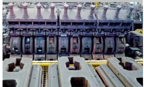
At the Vallourec & Mannesmann Tubes rolling mill, the Turck BL ident system ensures that only the correct roller cages are used for the batch. Page 20
