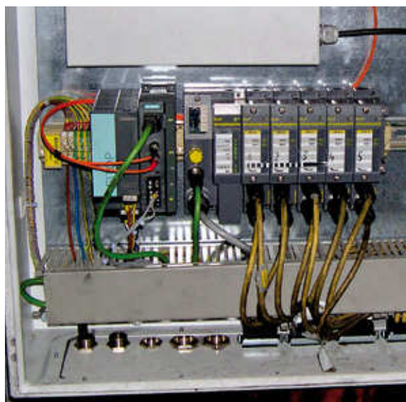
The gateway of the BL ident programmed in Codesys communicates with the operating computer
