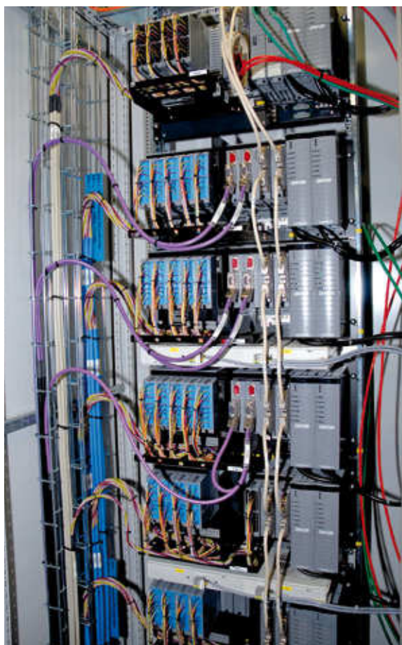
The redundant Profibus connection of the Yokogawa Centum VP control system increases availability
