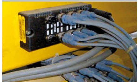
Turck's fully encapsulated BL compact I/O modules withstand the harsh ambient conditions in the paint shop of a Chinese car manufacturer. Page 30
