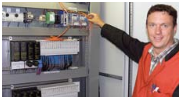
For Sasol's plant in Brunsbüttel, Germany, Turck delivered more than 30 excom remote I/Os.
